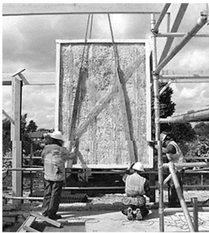
Figure 11. Loadbearing strawbale construction in Arizona, USA; [1].
