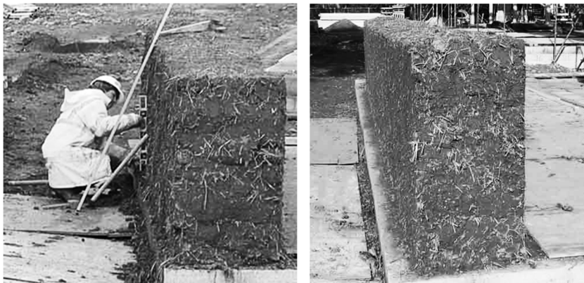
Figure 7. Cob wall construction at the Genesis Centre; [10–12].
