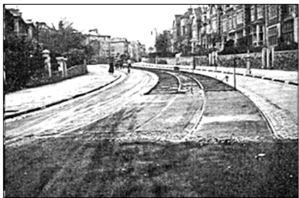
The three stages of track lifting on Redland Hill during 1982, as documented by S. Miles Davey.
