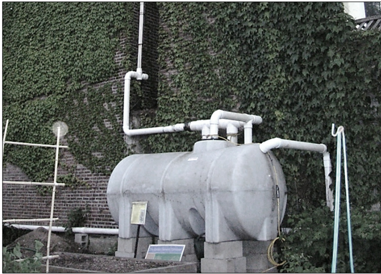
Plate 58. Rainwater harvesting and closed loop systems.
