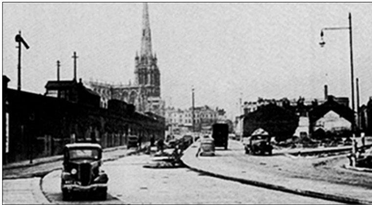
Taken on 28 October 1939, Redcliffe Way under construction. A gap had been created within the distant buildings to accommodate the new dual carriageway designed to cross the water. To the left, the railway sidings were positioned above a row of workshops, while one side of the newly constructed road had already been opened to traffic.
