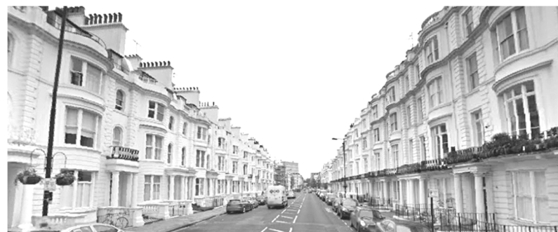
Figure 2. Gloucester Terrace, typical canyon view.
